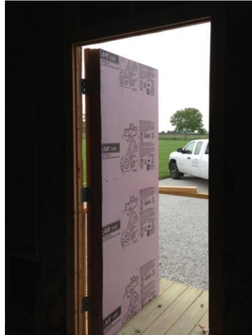
Figure 2-10. Enhanced Shelter door with XPS insulation attached.
