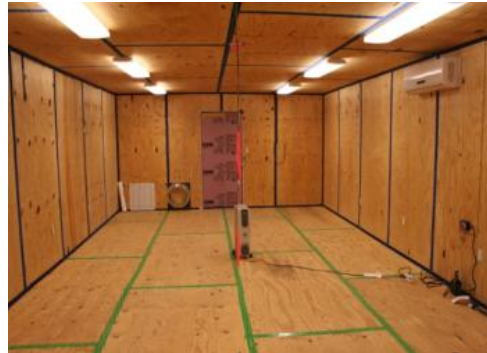
Figure 2-11. Unimproved and improved B-hut interiors: The inside of an unimproved B-hut (left) and a B-hut fully taped from the interior with air barrier tape (right).
