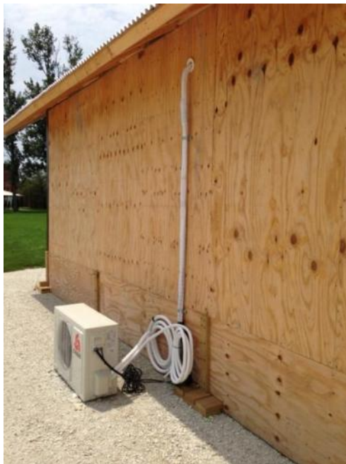
Figure 2-4. Chigo mini-split exterior condensing unit.
