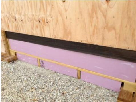
Figure 2-9. Enhanced Shelter skirting XPS insulation behind panel.
