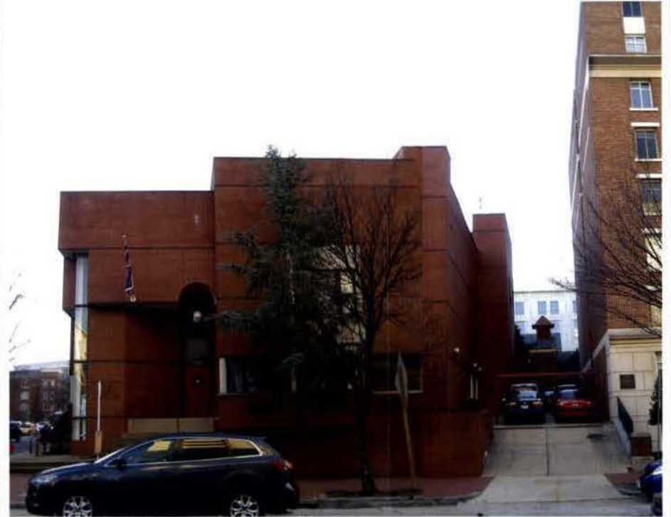
VIEW ALONG H STREET, NORTH ELEVATION
