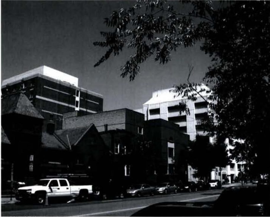
EXISTING HILLEL, SE VIEW
