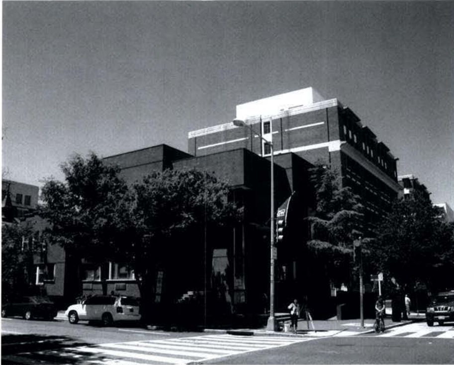
EXISTING HILLEL BUILDING
