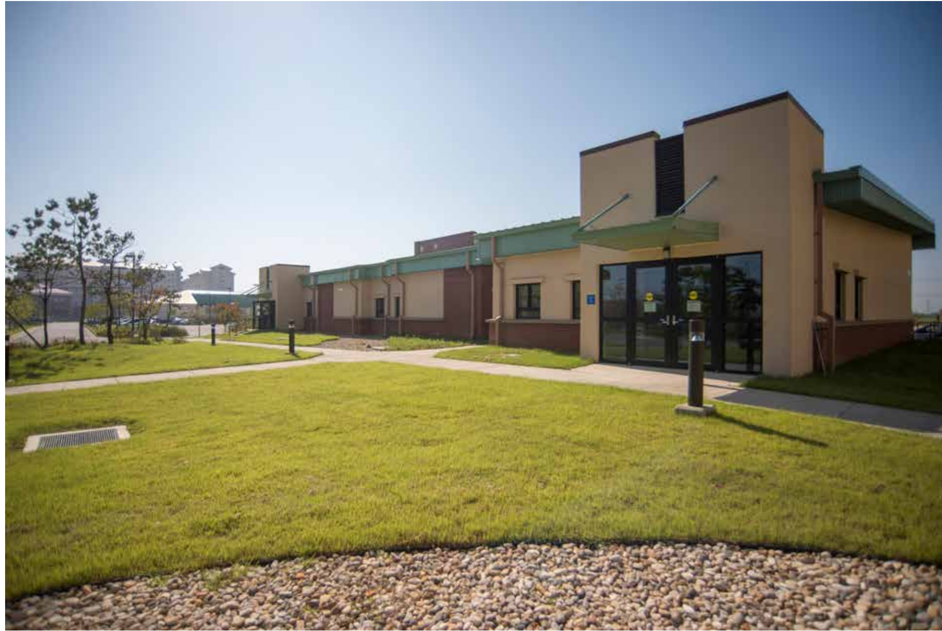
The Richard E. Cowan Post Office is located in building P-6809 between the Pfc. Ross A. McGinnis Warrior Zone and the Sitman Physical Fitness Center. This places it within walking distance for Soldiers living quarters in the newer areas of the installation. The post office is open Monday to Friday from 11 a.m. to 1 p.m. for outgoing mail services.
