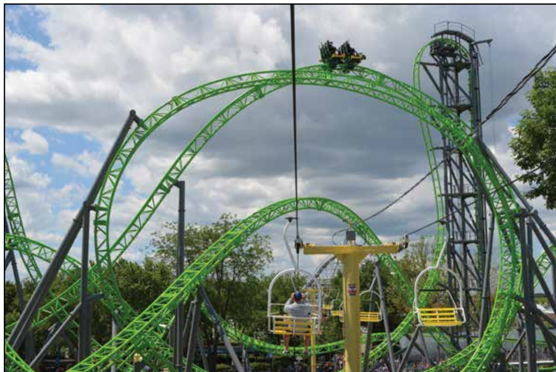
Adventureland's new Monster posed unique design challenges for Gerstlauer — resulting in a track layout that goes over or under the park's sky ride eight times and sees sky ride riders pass through four of the five inversions. COURTESY ADVENTURELAND PARK
