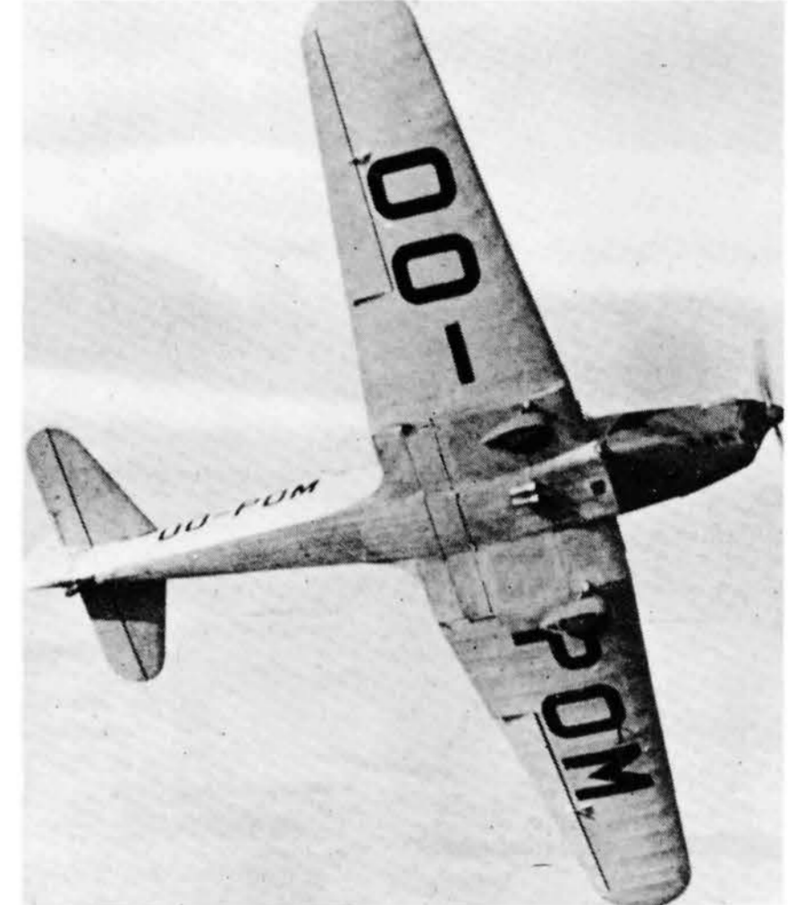
Right: OO-POM from the underside shows the small span centre-section flaps set forward from the trailing edge. (Aeronautics via Jack Meaden) Below: When OO-POM arrived in Britain post war it had a new hood with deeper transparencies and a partial windscreen for the rear cockpit. On the right side it wears a Topsy Trainer motif, the name used originally for British built Topsy Bs pre-war. (Fairey via Jack Meaden)
