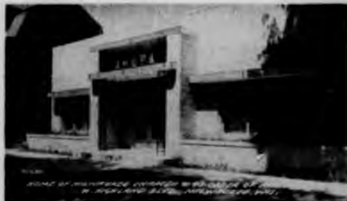
MILWAUKEE AHEPA — Headquarters of Milwaukee Ahepans is the above modernistic Ahepa Hall located at 3208 West Highland Boulevard in the Wisconsin metropolis. Milwaukee Chapter No. 43 meets there on the first and third Wednesday of each month. When in Milwaukee, be sure to visit the Ahepa Hall. A welcome awaits you.
