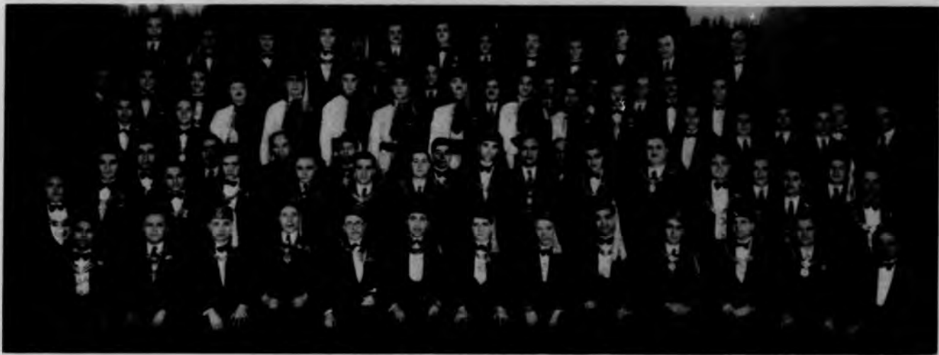
Six New Jersey Chapters Hold Combined Installation at Trenton
