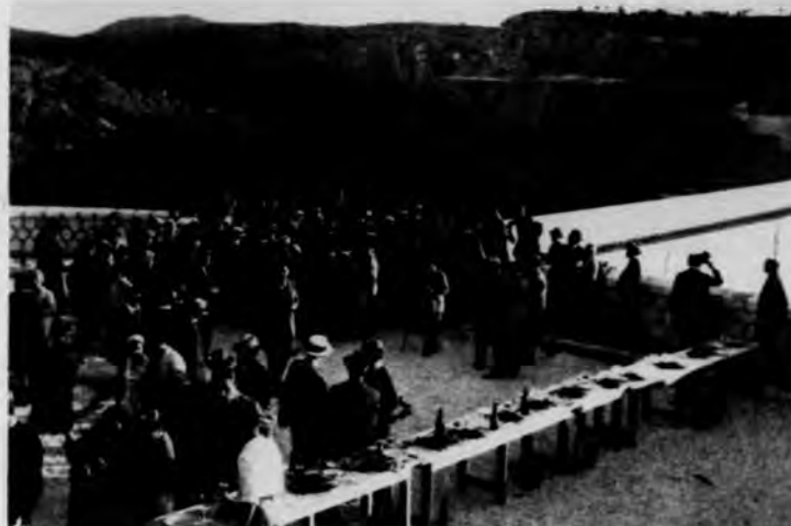
Inaugural ceremony held at the Marathon Dam, at the completion of the new water supply system of Athens, attended by officials of the Greek Government and Ulen & Co.
