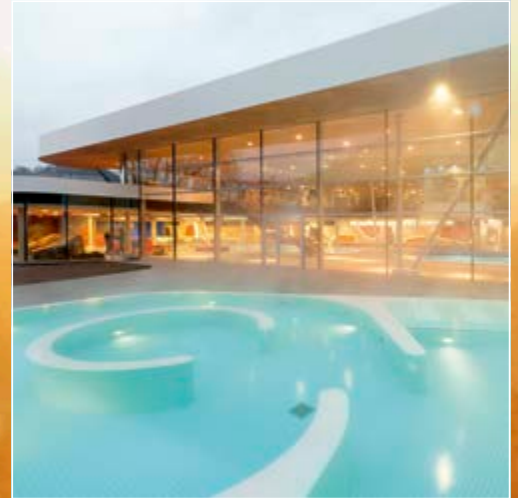
Ideal for the spa area Ems Thermal Baths, Bad Ems, Germany / Architect: 4a Architekten, Stuttgart / Photo: David Matthiessen
