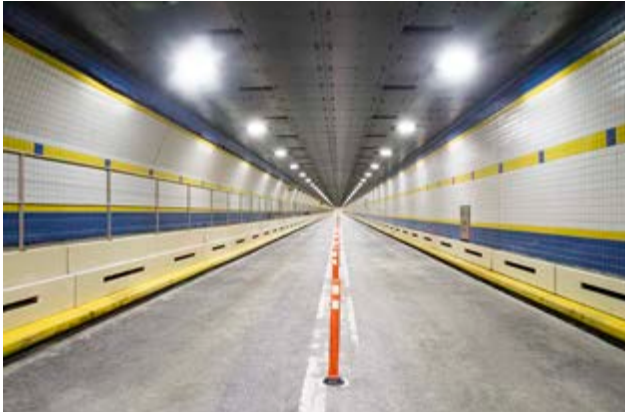
Even cleans the air in tunnels Hugh L. Carey Tunnel, New York, USA / Architect: HAKS, New York / Photo: Titus Kana
