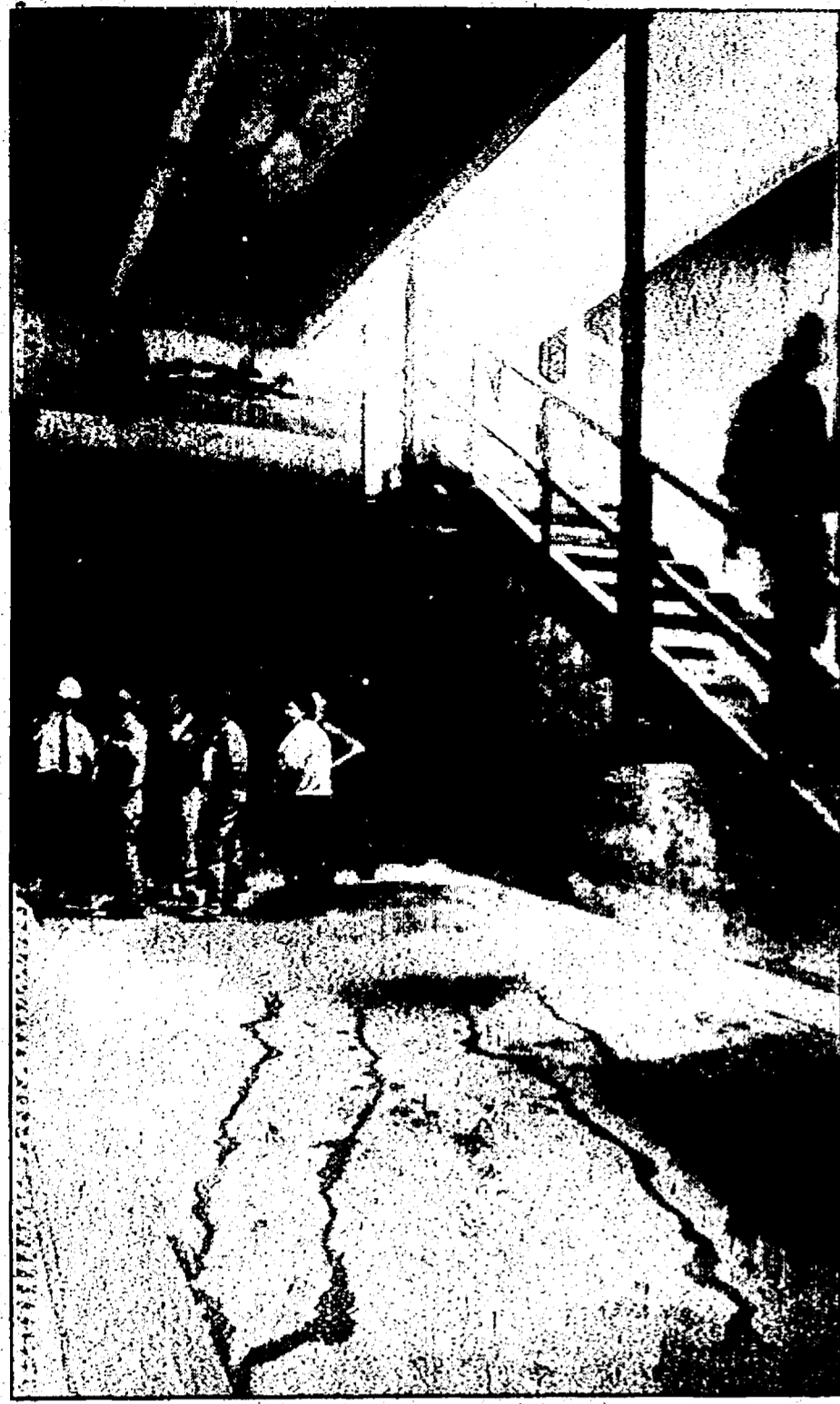
Down under: Chuck Lemont, resident engineer for Wade-Trim Associates Inc., leads guests around one of the water holding tanks at the CSO Basin in Inkster.
