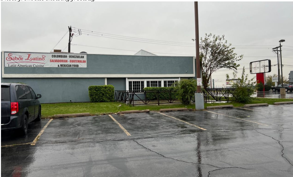
Adjacent property south of site
