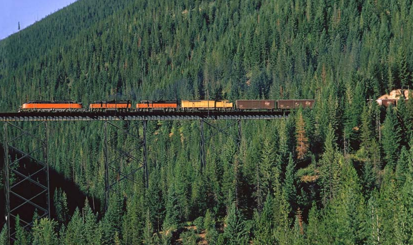
In typical fashion, a Milwaukee Road Little Joe electric teams up with two run-through GP40s and an FP45 hauling freight east over St. Paul Pass, Idaho, in 1970. George W. Hamlin collection
