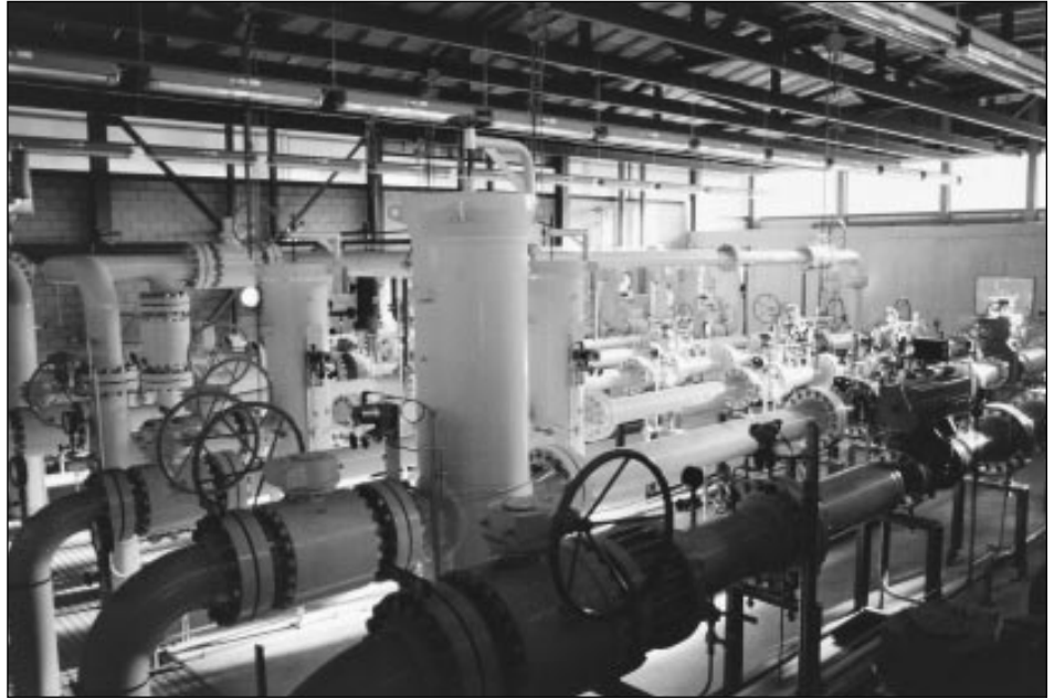
Soft-Concept used National Instruments BridgeVIEW to create a PC-based SCADA system to monitor this gas pipeline system.
