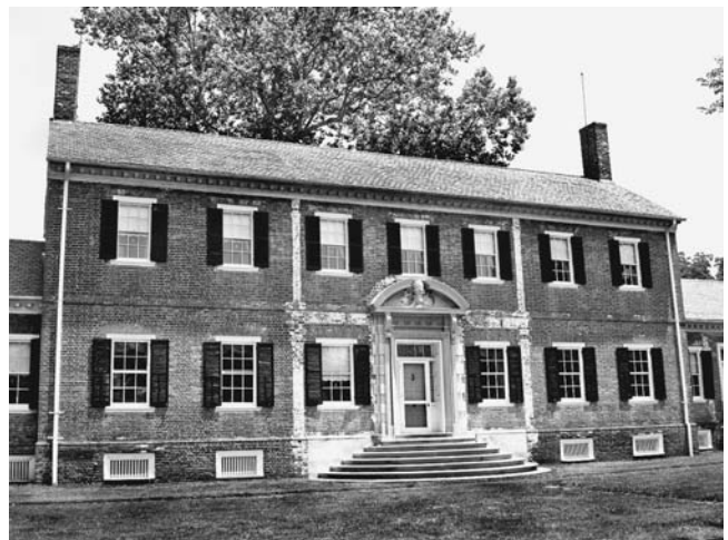
Chatham manor house. Photo by R. E. Guiley.
