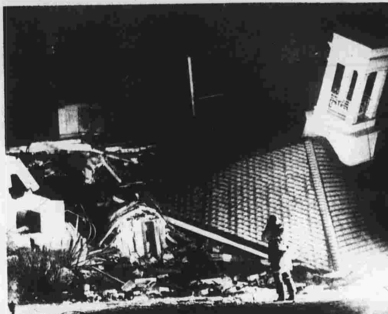
Roof of the two-story Shaker Heights police station rests on the ground after an explosion virtually demolished the building. At least 15 persons were injured. (AP Photofax)
