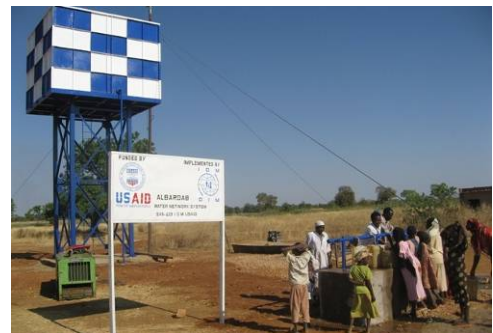
Photo III 1: Water Distribution System Al Bardab, Southern Kordofan
