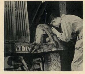
T-3 Bruce Warner welds the cracked fender of a German personnel carrier received at Aberdeen.
