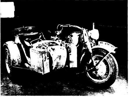
A side-car version of the BMW (Bayerische Motoren Werke) which has a unique motorcycle feature—a reverse gear. Unlike American models it has a hand clutch. This is as good as any motorcycle in the world.
