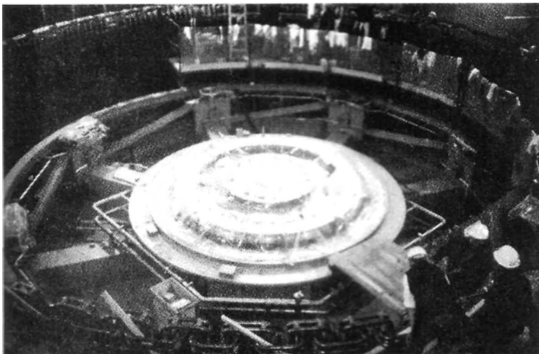
A generator under construction at La Grande 1.
