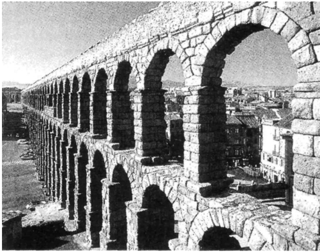
Roman Aqueduct, Segovia, Spain
