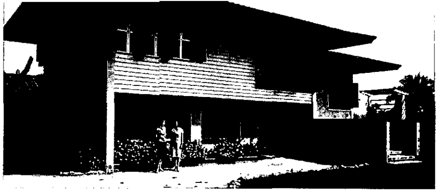
MIXED STYLES characterize tidy building which serves as Peace Corps headquarters in Bangkok.
