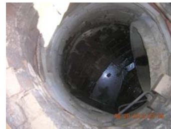
View inside Smith Street manhole
