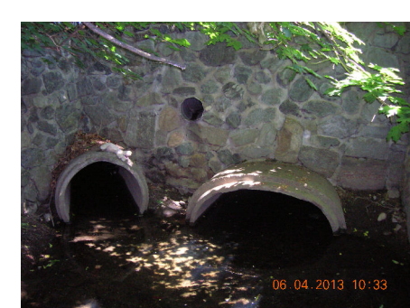
...and flows out the outfalls...
