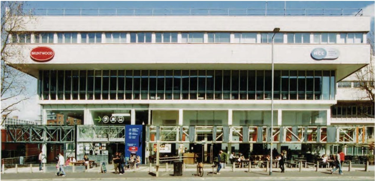
Figura 3. Manchester, Bruntwood's refurbishment of the former National Computing Centre, 1964. Fotografía: Richard Brook. http://www.mainstreammodern.co.uk/ [Consulta: February 23rd 2017].
