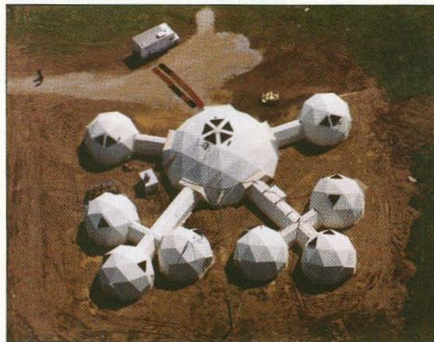
Photo A. Aerial shot above Moonbase America.
