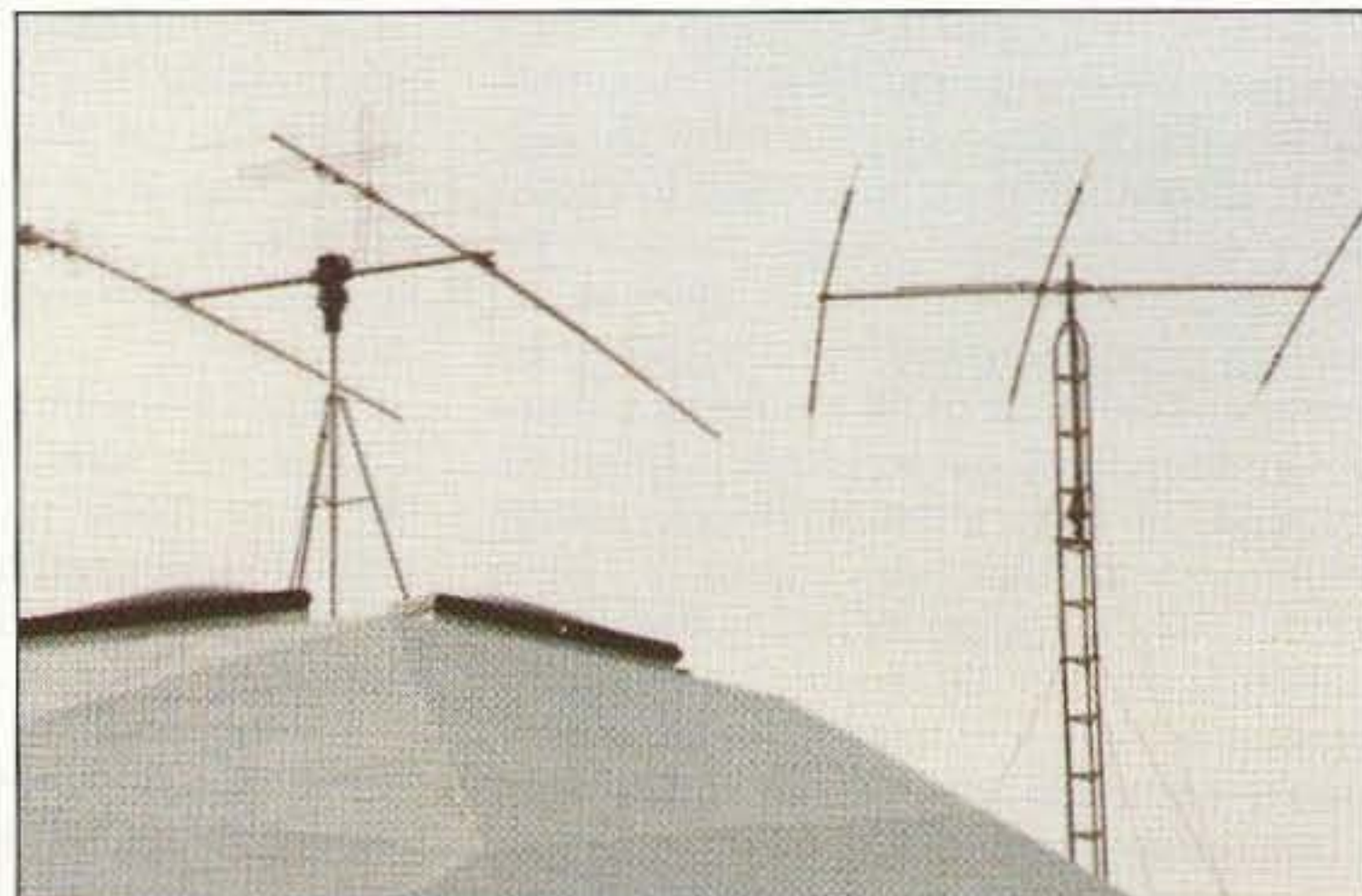
Photo B. Satellite tracking antennas (on the left) on top of the main dome of Moonbase. To the right is a 3-element triband HF beam on a 40-foot tower.
