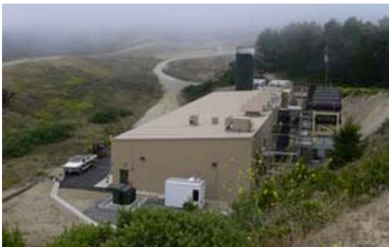
Figure 2. Ox Mountain's Landfill Gas to Energy Facility in Half Moon Bay, CA
