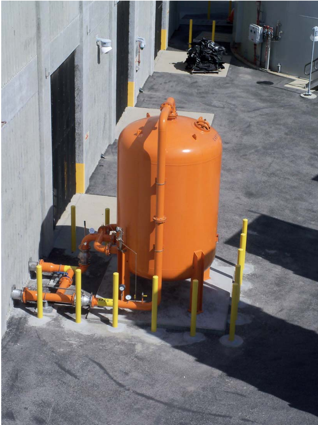
Figure 2-3: Digester Gas Cleaning System
