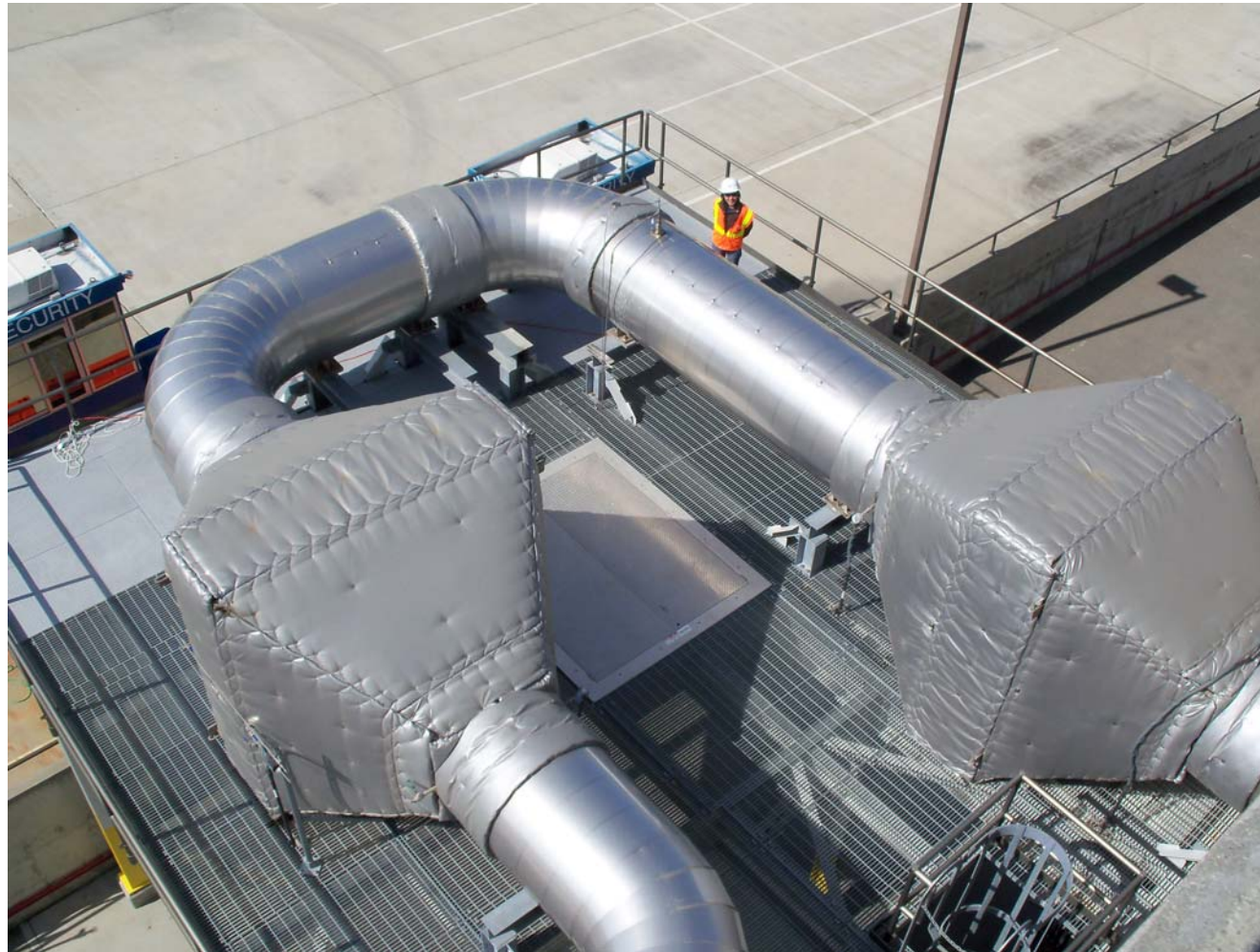
Figure 2-4: Cat Ox/SCR Platform Installation
