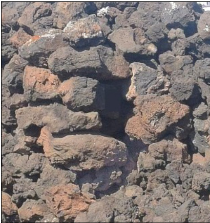
Fig. 8 - Multiplex soul-hole, upright sized oriel type, stones partly stacked, centered in the supporting wall (Pto. del Carmen, Lanzarote) [Photo: H.-J. Ulbrich].
