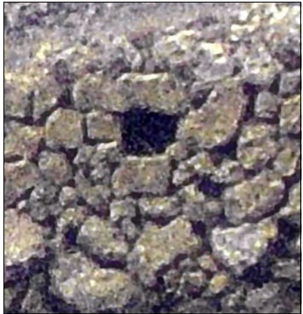
Fig. 13 - Multiplex soul-hole, big lintel + threshold, nearly quadratic tubus in upper half of the wall, help of a mason / see also figs. 14/19 (Tinajo, Lanzarote) [Photo: H.-J. Ulbrich]
