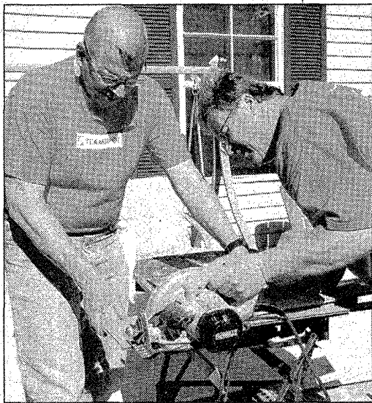
Working on the home are Tom Keyser (left) and Doug VanGordon.
