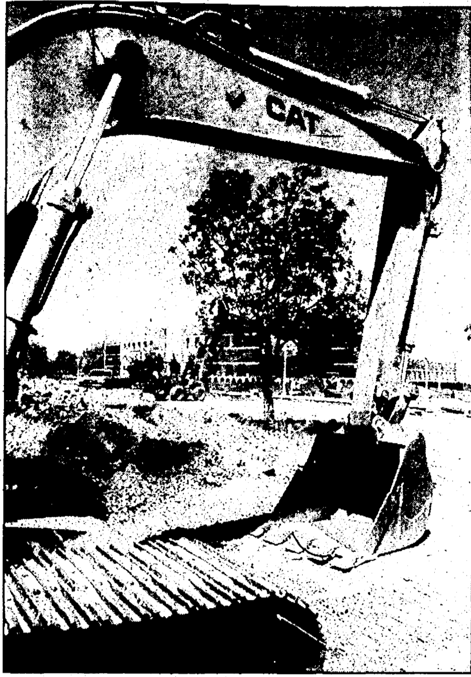
New asphalt: Contractors from Nagle Paving Co. of Farmington Hills are expected to wrap up construction by mid-July of an expanded parking lot at Schoolcraft College adjacent to the McDowell Center and Grote Administration Building. Asphalt is expected to be poured next week. Approximately 60 parking spaces will be added for faculty, staff, students and visitors as a result of the $388,214 project.
