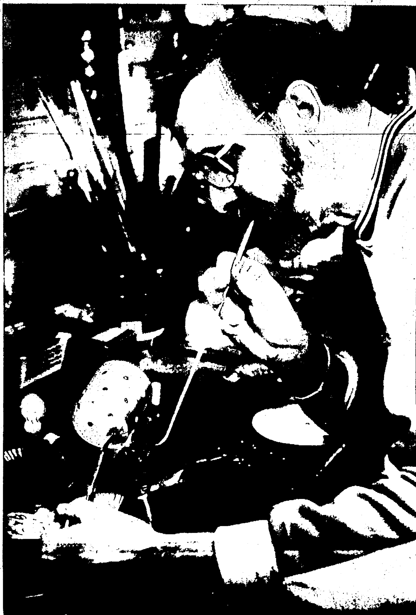
Bob Horwood uses handpowered tools from a mid-1800s tinshop to create a tin object. The purchase included an old log with hollowed-out bowl shape forms that the tinsmith used to hammer, shape and round the tin.
