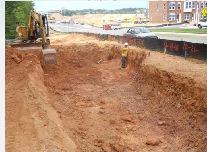
Excavation performed from outside the footprint of the permeable pavement area
