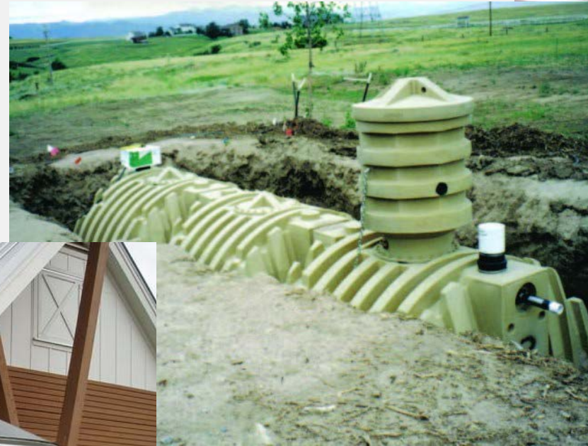
Below-Ground Cistern – PermaDesign
