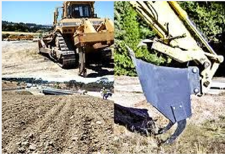
Tillage and ripping done to scarify native soil
