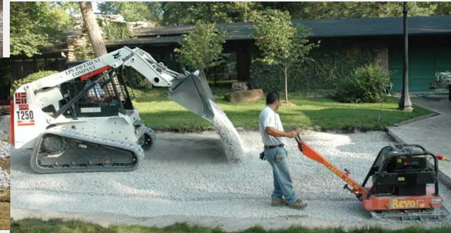
Compaction of aggregate base layer often done using vibratory roller and compaction done every 6-inch lift
