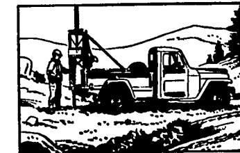
Mobile drill, mounted on the 'Jeep' Truck, is operated from the truck engine, through power take-off.
