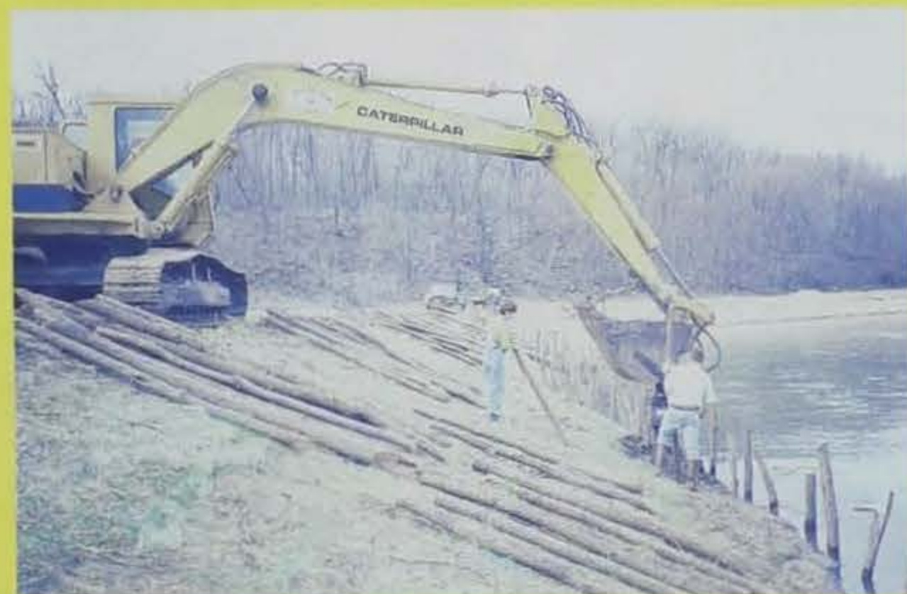
Streambank stabilization along the Volga was not easy for the Kerns. Planting willow posts along the streambank (left). A before (top) and after (bottom) look at the Kerns' Volga River streambank.
