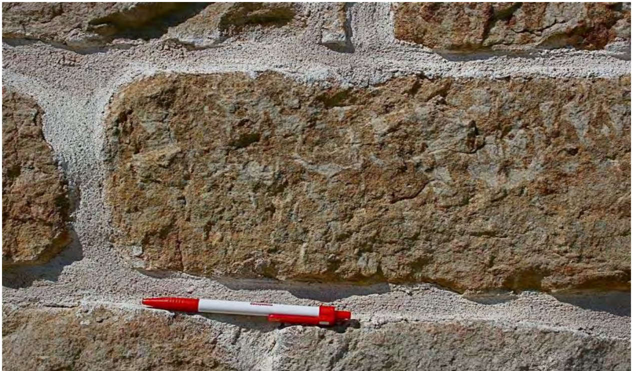
Fig. 5 Typical building stone in walls of the Old Stone Mill at Delta, built in 1810. This block, like most others in the outer walls of the mill, displays two varieties of distinctive trace fossils. Colour contrasts outline abundant vertical tubular burrows of Skolithus and several U-shaped burrows of Diplocraterion .
