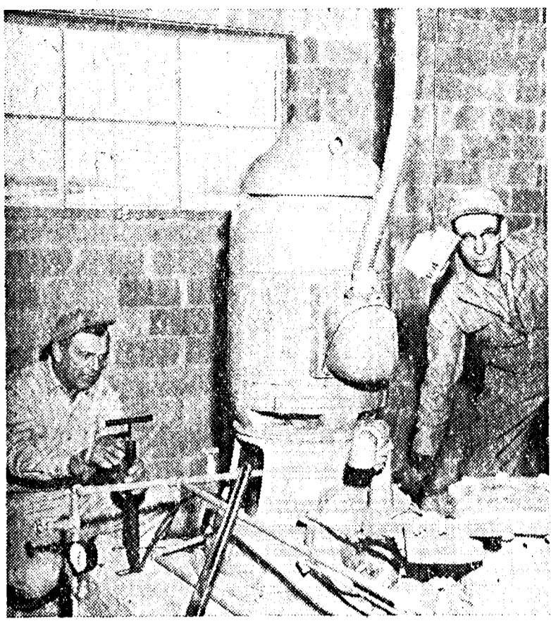
Well heads where water starts . . . City Employees Wayne Pierce and Bill Beard make last minute adjustments on the 700 gpm. pump that draws the water some 180 feet to the surface.
