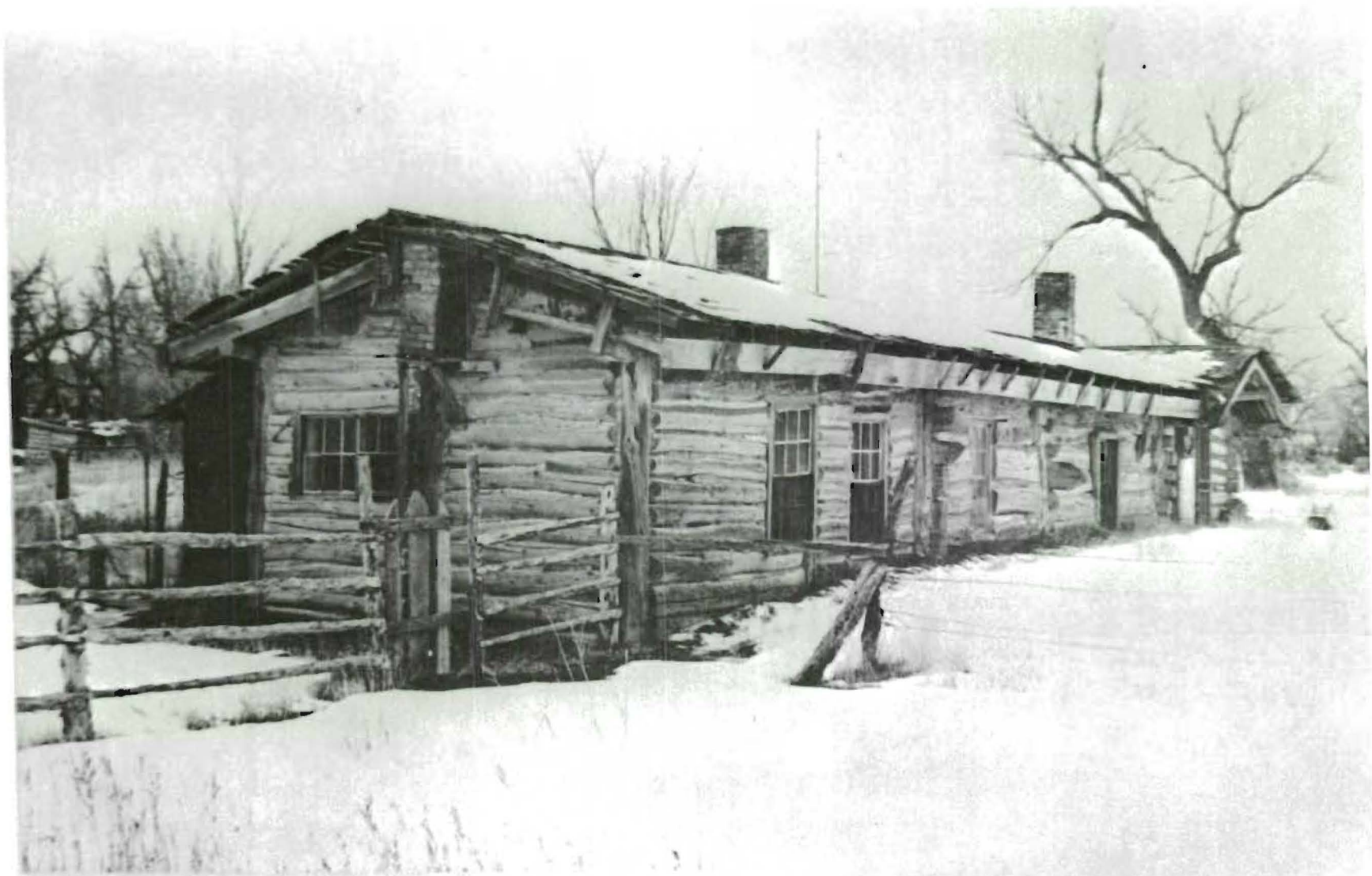
Photograph of the "Deacon" Wade ranch home built in the 1880's, located about 12 miles south of Medora. The portion in the foreground is a part of the original structure. (Photo by Richard Weeder, February 1961.)
