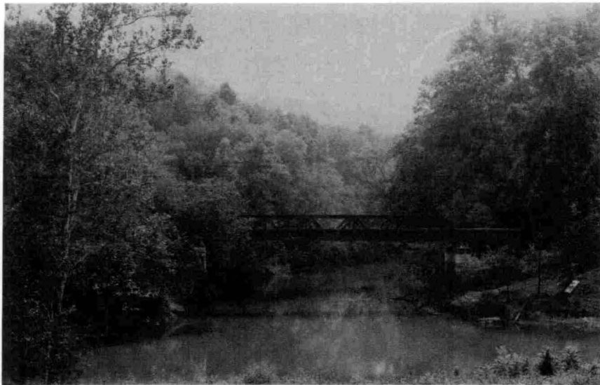
Railroad Bridge over Birch River at Elk River junctior
