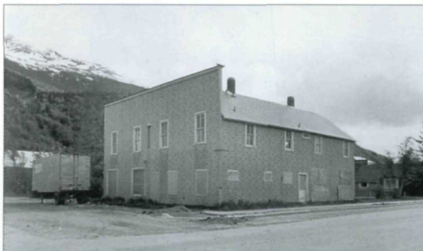
The Moore Block building, constructed circa 1897, has seen many uses and a variety of modifications in its history. This circa 1975 view shows the building much as it appears today—its wood siding covered with asphalt brick sheathing and its windows covered in plywood. Photograph courtesy of NPS Alaska Support Office.
