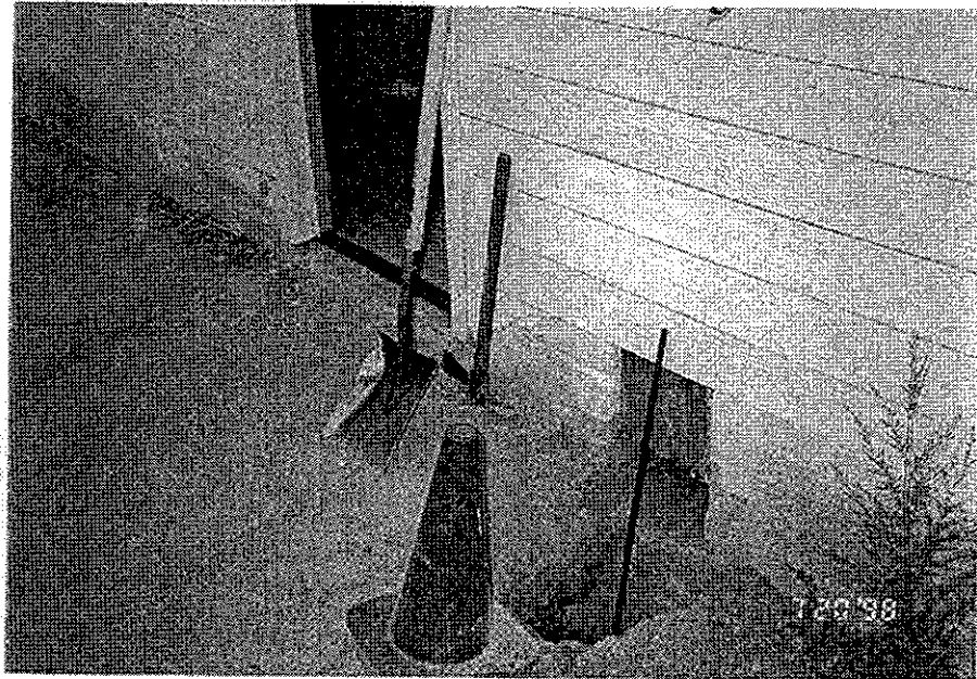
Photo No. 13 Bottom of South Column at Grids A-4
