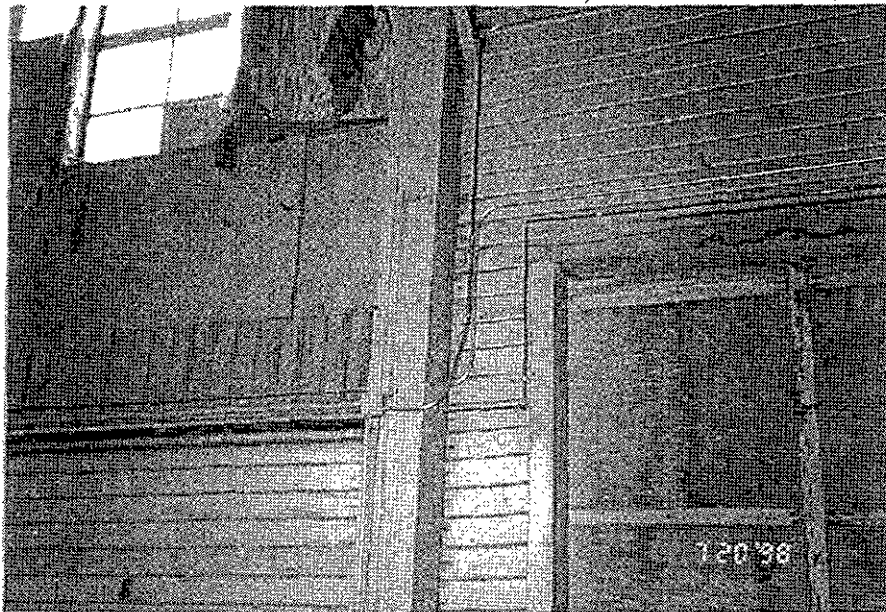
Photo No. 6 Wall Openings on Grid A at Grid 7
