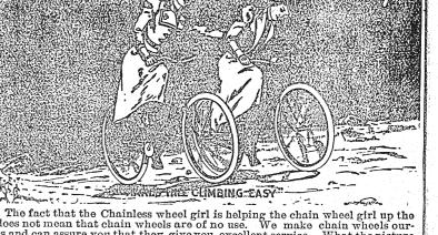
hill does not mean that chain wheels are of no use. selves and can assure you that they give you excellent service. What the picture shows is that the Chainless is the better hill-climber. Why is this? Simply because the bevel-gearing cannot be cramped or twisted under the extra strain. This same uniformity of action makes the Chainless an exceptionally easy run-ning machine under all conditions of riding.
