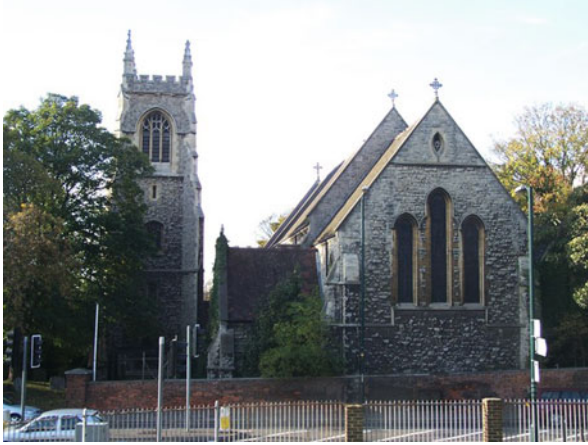
Fig. 1 St Mary's Church (1884–1887), Chatham (Kilic 2012)
