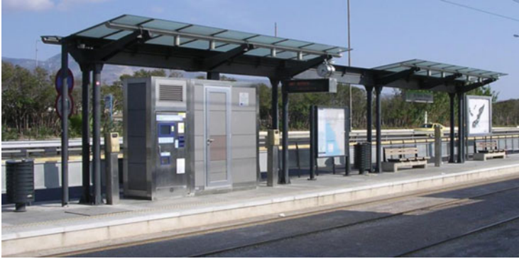
Fig. 1 Shading device on a side-way boarding platform, in the station “2nd Agiou Kosma”
