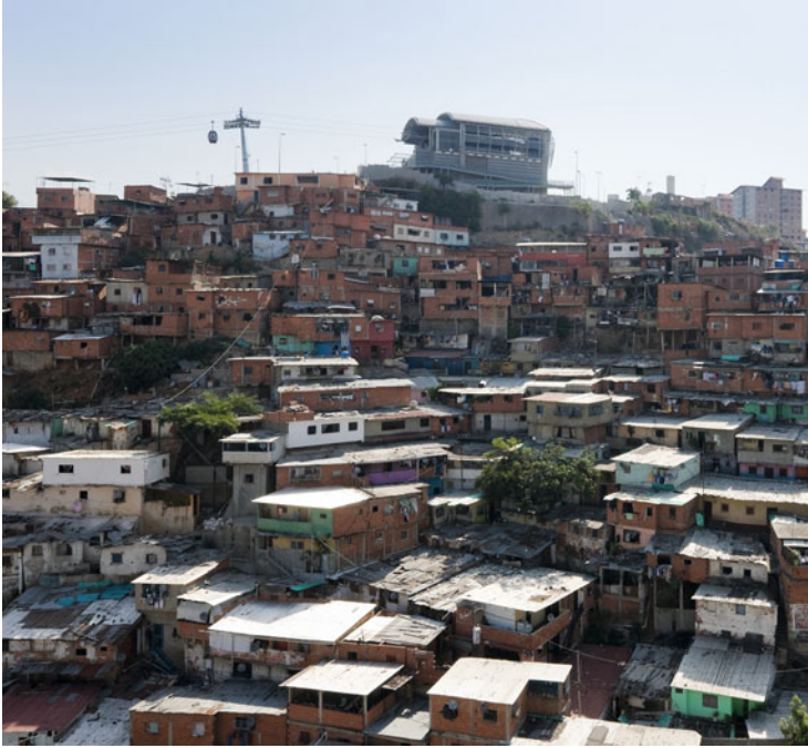
Fig. 6 El Mangito station sits along the ridge of the San Agustín neighborhood (Iwan Bann)
