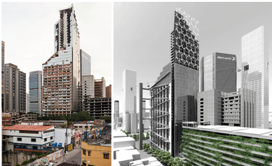
Fig. 10 (Left) Torre David today, a vertical slum without elevators, air conditioning, and any formal infrastructures. (Right) The tower transformed through micro-scale interventions that have improve living conditions and foster urban communities (Urban-Think Tank Chair/ETH, Zurich)
