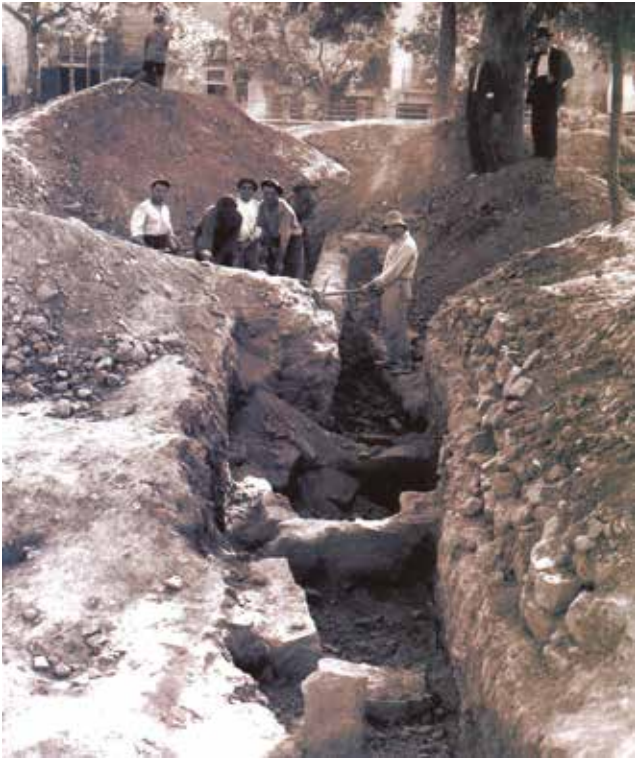
Fig. 1. Excavation of the Plaça del Vell Pla (1993) by Josep Colominas of the IEC.
