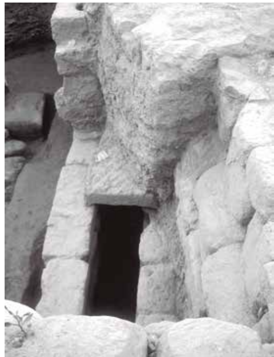
Fig. 9. The sewer drain along the western edge of the cardo maximus of Ilerda, near the city's public baths (photo: I. Gil).
