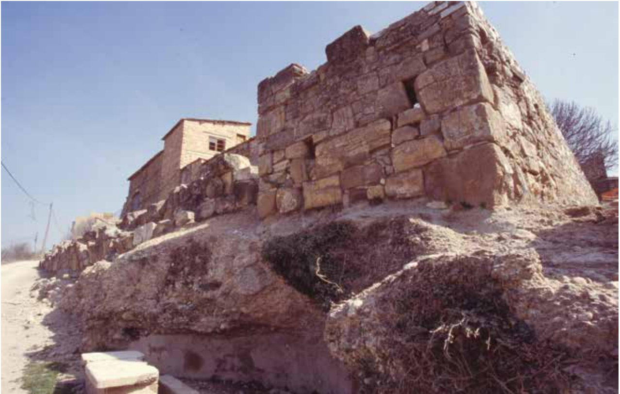
Section of the wall of the Torreta Street (photo: S. Martínez).
