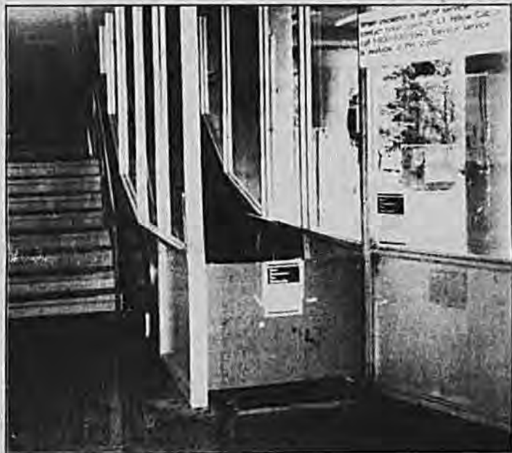
NEW ESCALATORS will be installed at the Hicksville railroad station as part of the LIRR Capital Improvement Project. The four-month project is scheduled to begin on August 24 and continue until Christmas. Train service should not be affected. Photo by JW Garger
