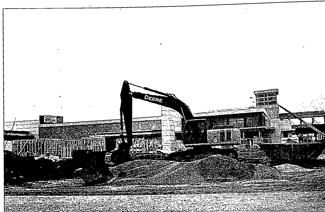
The Des Plaines Casino near Park Ridge is now named Rivers Casino. Construction is still going on. The casino will be located on the corner of River Road and Devon Avenue. | Tamara Bell-SunTimes Media
