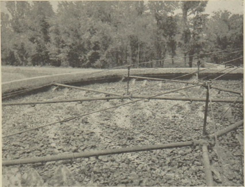
FIGURE 3.—Portion of filter surface, Camp Fannin, Texas, showing absence of growth in some areas caused by filter fly larvae.
