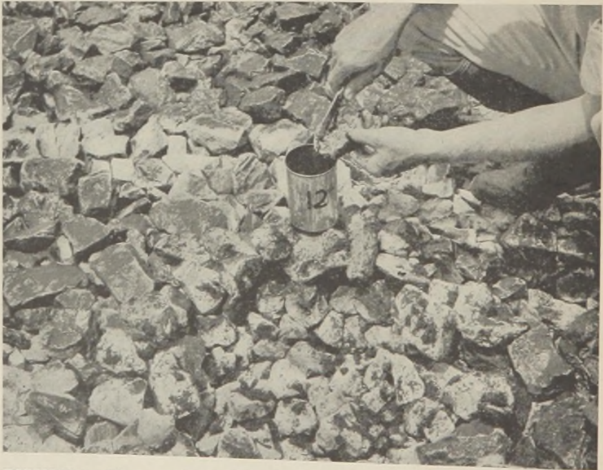
FIGURE 2.—Close-up view of trickling filter surface at Camp Fannin, Texas, showing stones denuded of growth by filter fly larvae. Note heavy infestations of larvae in foreground.
