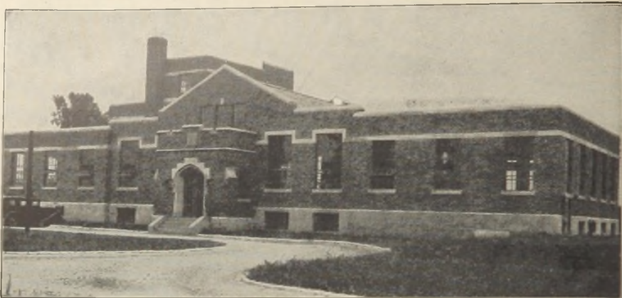
Water Softening Plant, Fremont, Ohio
