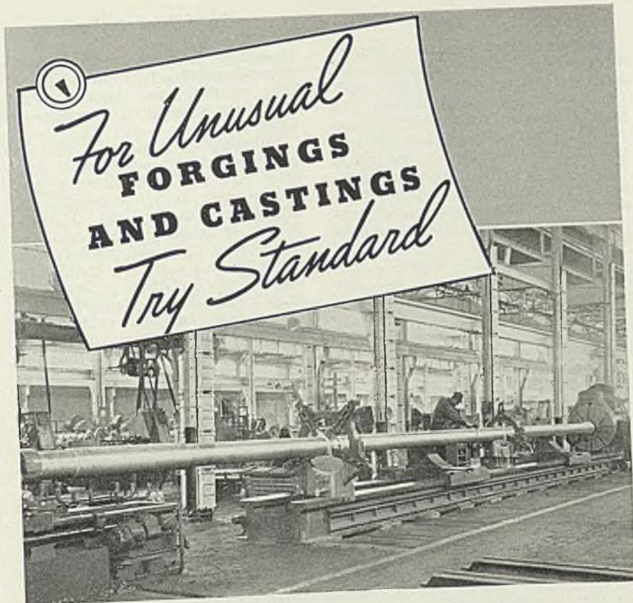
● Shaft 57 feet long, largest diameter 11 $\frac{3}{4}$  inches, weight 17,300 pounds — forged and rough machined by Standard Steel Works Company.
