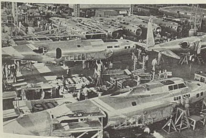
■ After being assembled in a series of steel jigs in another section of Boeing Aircraft Co.'s plant at Seattle, these B-17B bomber bodies take their place at the start of final assembly line. As each body receives its wings, on which landing gear has already been installed, it is rolled forward in the line. Body in middle of picture is just being lowered by overhead cranes to its place on assembly floor
