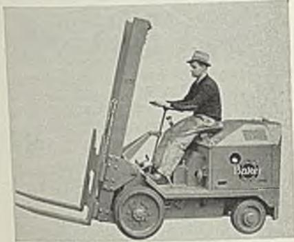
cylinder Hercules industrial gasoline engines designed for continuous operation at high power output and rubber mounted to reduce vibration. Heavy-duty industrial-type transmission and clutch are used, gearbox providing two speeds forward and two reverse. Hydraulic brakes on drive wheels and all controls of automotive type are provided.
