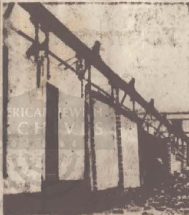
MONORAIL moves prefabricated cement walls and floors to construction sites of apartment buildings in Bucharest.
