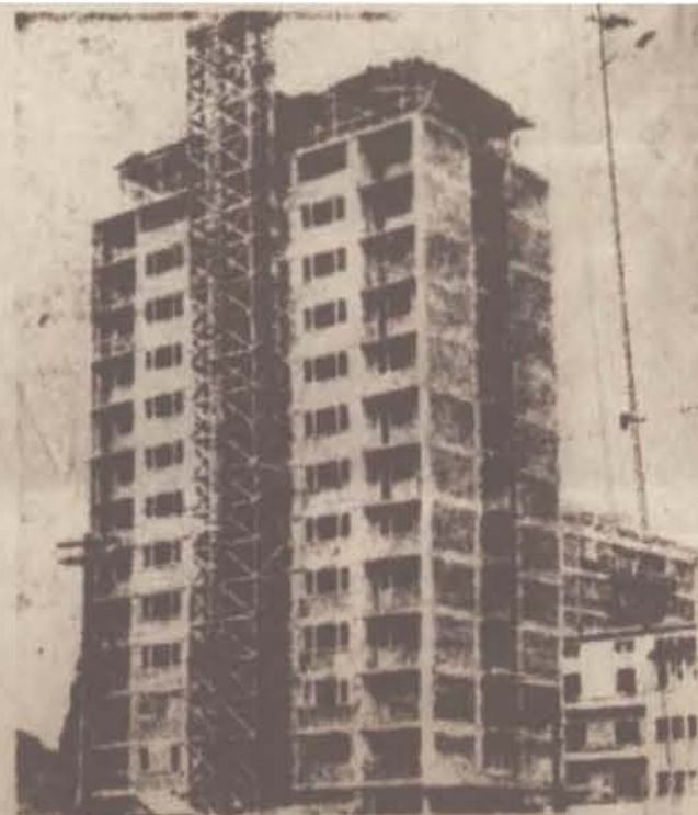
SIXTEEN-STORY-HIGH apartment building in Bucharest replaced a ramshackle housing development.
