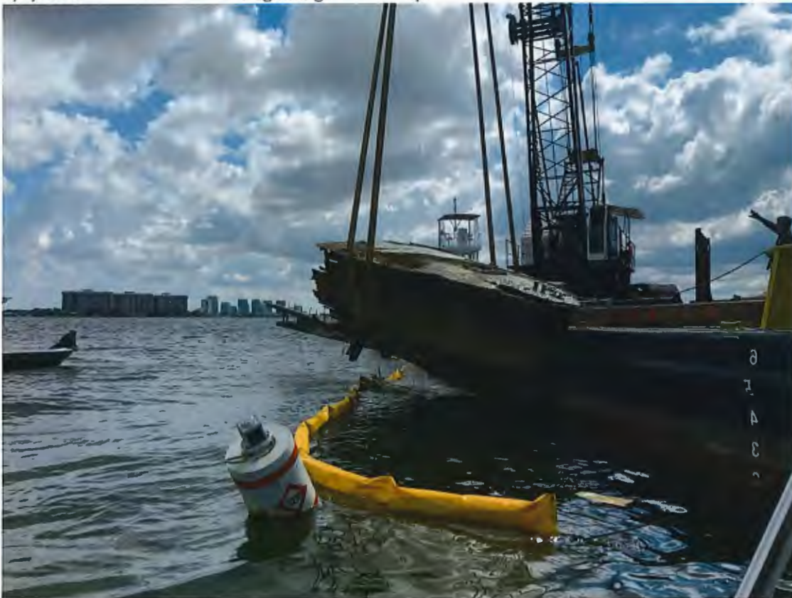
10/16/2019 – Vessel removed in pieces.
