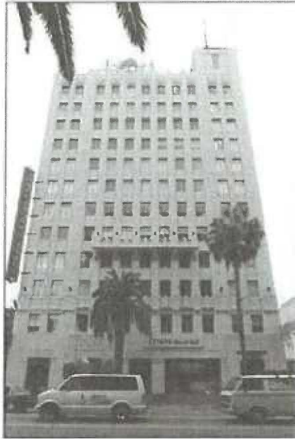
Photo 3: Bank of Hollywood / Equitable Building, south elevation, view north (Chattel 2014)
