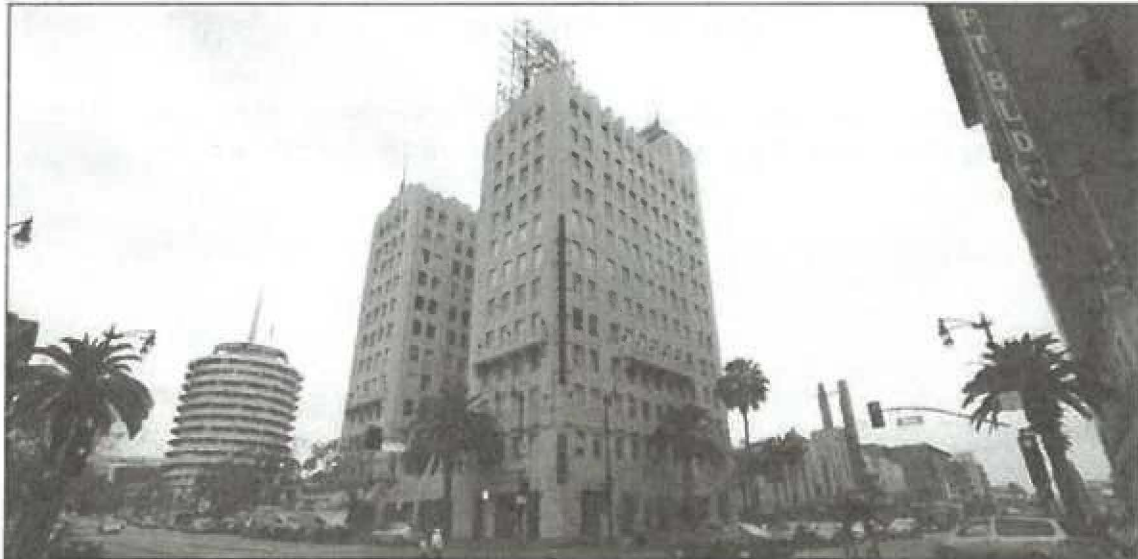
South and west elevations, view northeast (Chattel 2014)
