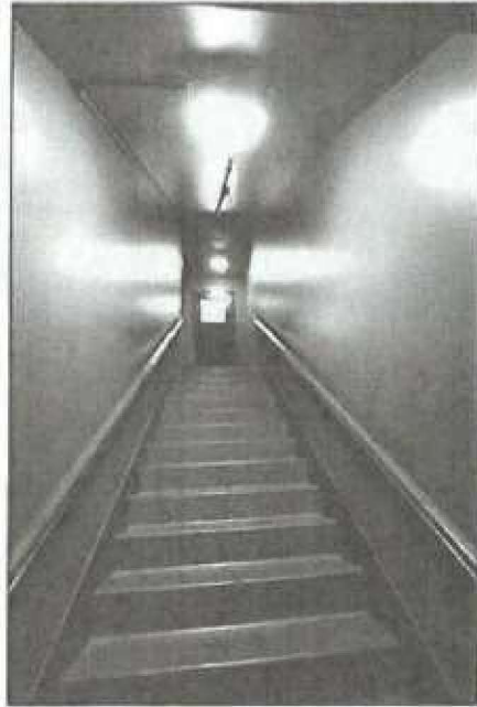
Photo 27: Bank of Hollywood / Equitable Building, typical upper floor staircase (Chattel 2014)
