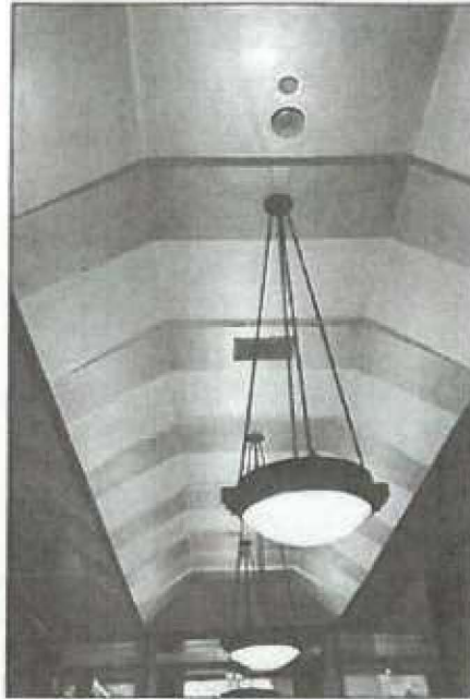
Photo 19: Bank of Hollywood / Equitable Building, main lobby, ceiling detail (Chattel 2014)
