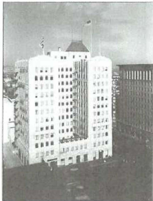
Image 10: c. 1931 photo of north and west elevations, view east (LAPL)
