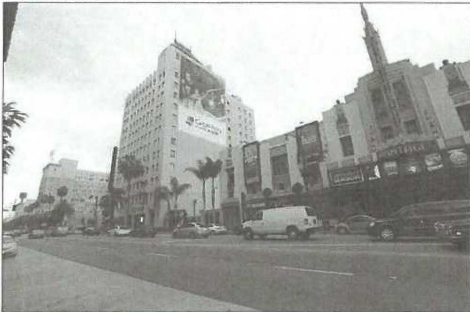
Photo 12: Bank of Hollywood / Equitable Building, south and east elevations, view northwest (Chattel 2014)
