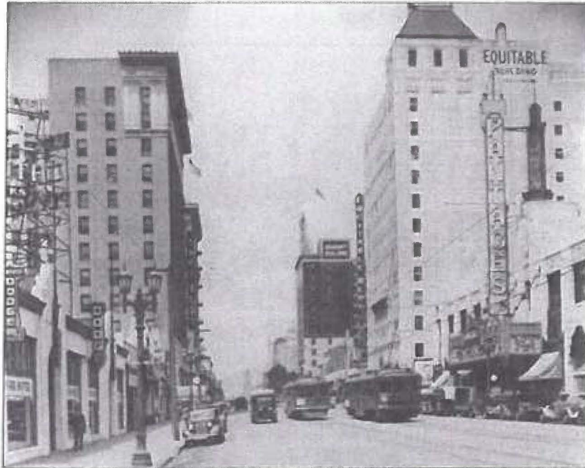
Image 21: 1936 photo of south and east elevations with Hollywood Boulevard development in foreground, view west (LAPL)
