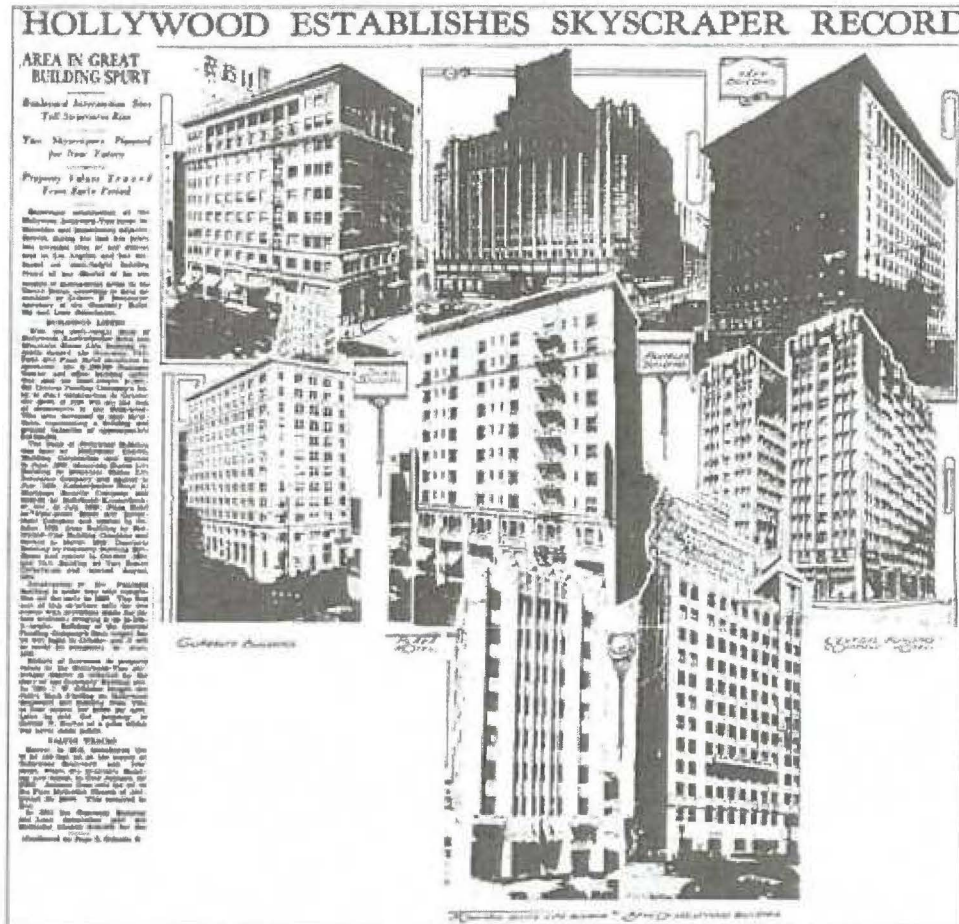
Image 3: 1929 article with photos of new Hollywood buildings, including subject property at lower right corner (Los Angeles Times)
