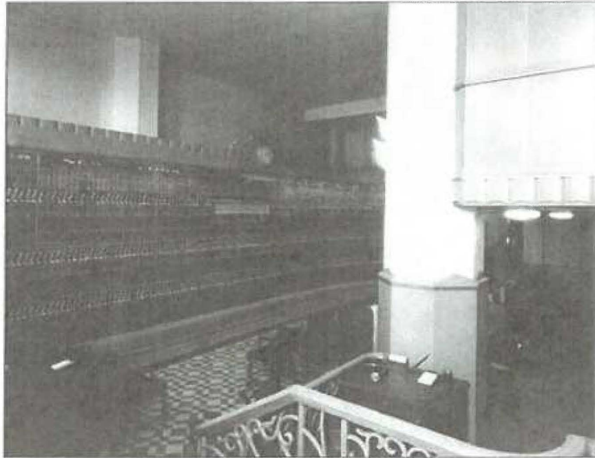
Image 17: 1932 interior photo of brokerage room (LAPL)
