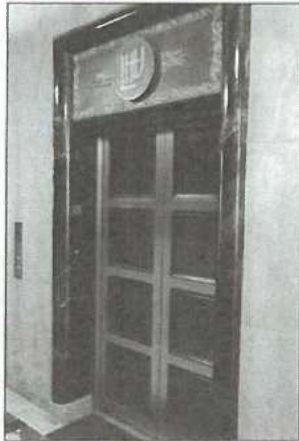
Photo 20: Bank of Hollywood / Equitable Building, main lobby, elevator detail (Chattel 2014)
