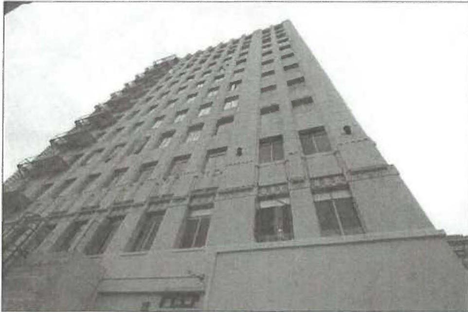
Photo 11: Bank of Hollywood / Equitable Building, north elevation, view south (Chattel 2014)
