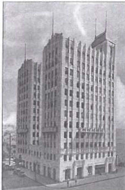
Image 6: 1930 rendering of south and west elevations, view northeast, note addition behind original tower to create U-shaped building (LAPL)
