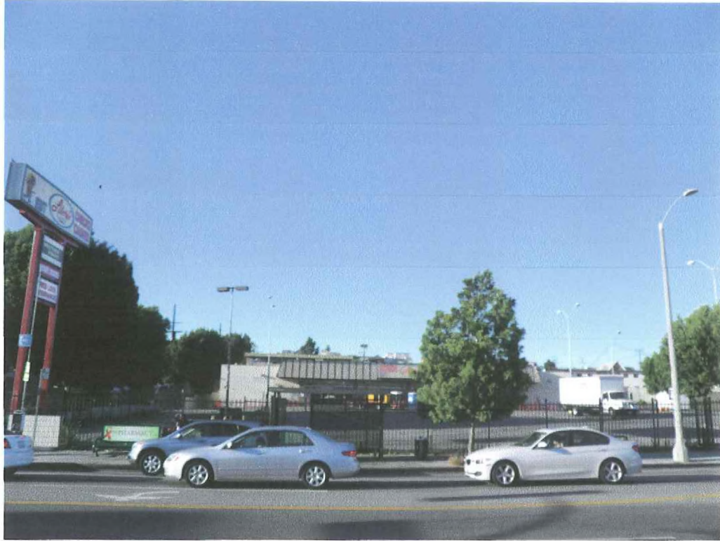
6. Site view from southern side of 3 rd Street.
