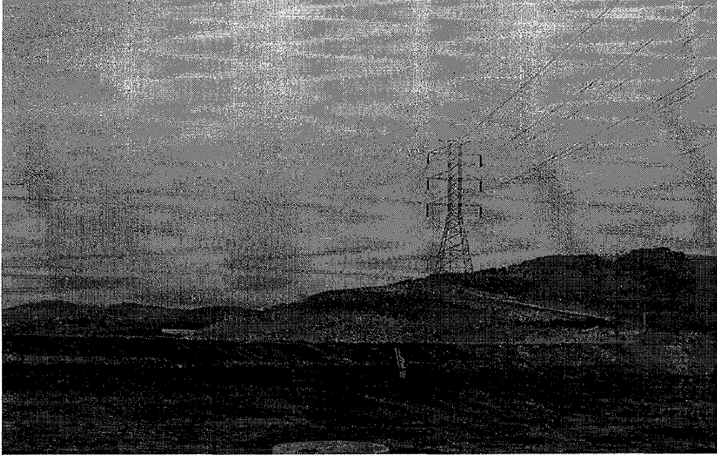
7. View of transmission tower on Parcel 3.
