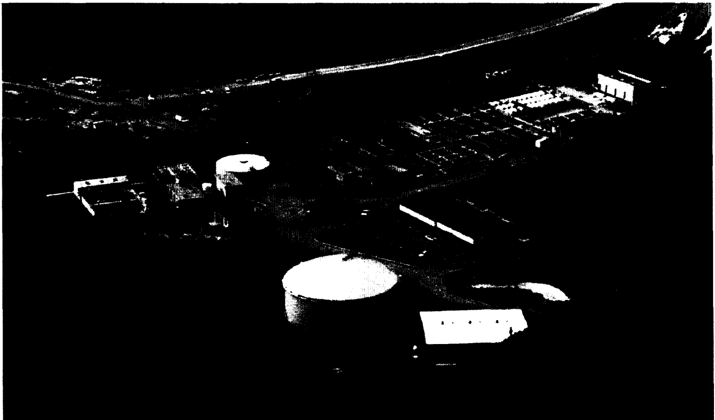
Overhead view off the Coastal Treatment Plant and Advanced Water Treatment Facility.
