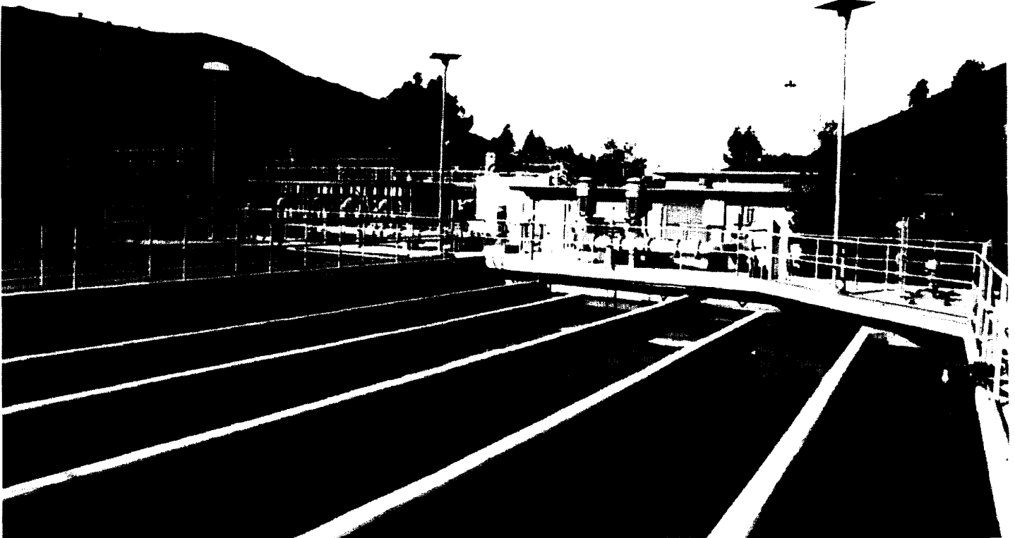
Wastewater is given tertiary treatment at the District's Advanced Water Treatment facility prior to use for irrigation and other non-domestic purposes.
