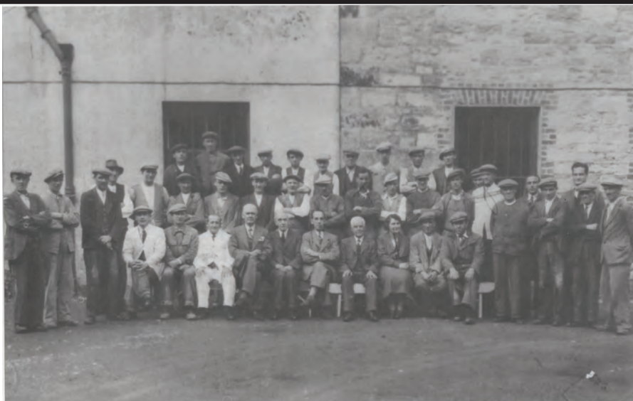
Lodge Mill Workers 1939/1940
