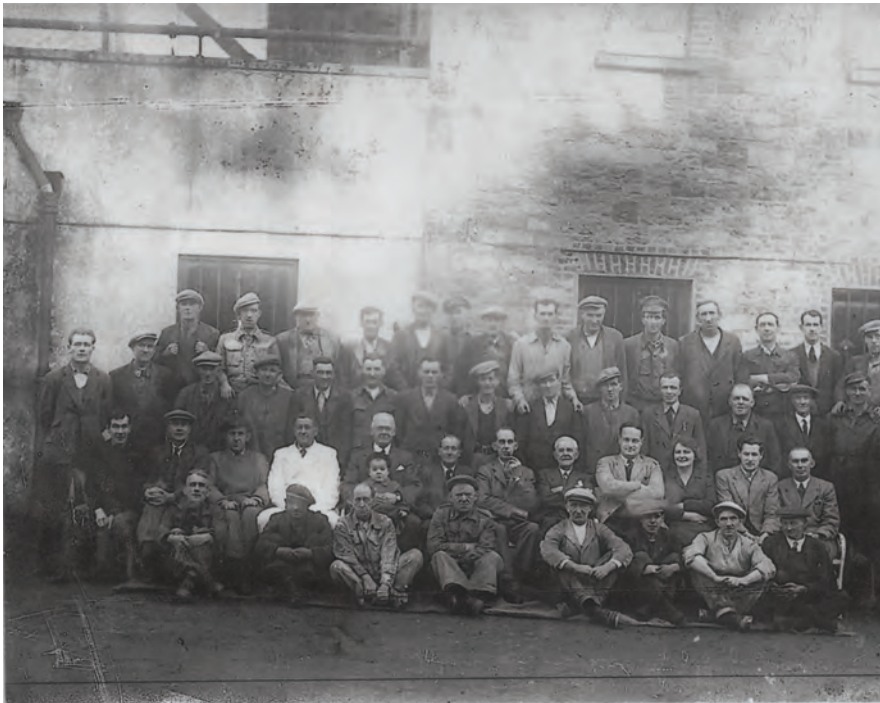
Lodge Mill workers 1947/48
