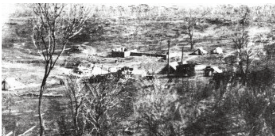
The Camp at Wilgie Hills with unfinished H-shaped building in centre of picture
